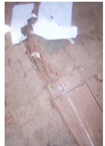
Girls dormitory termite damage of flooring
